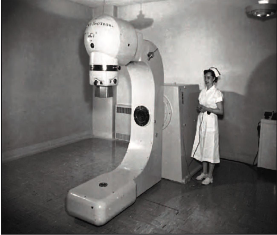
Figure I-B-1. Ontario Cancer Institute's X-otron cobalt-60 unit. (Reprinted from Fig. 7.1, p. 261, The Modern Technology of Radiation Oncology, Volume 2 , J. Van Dyk (Ed.), with permission from Medical Physics Publishing.)
